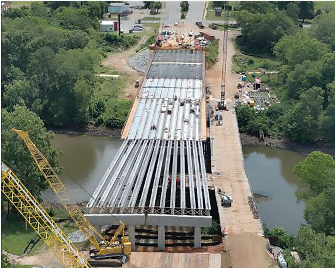
The new U.S. 82/State Route 520/Oglethorpe Boulevard bridge in downtown Albany is about 68% complete and projected to open this fall.
