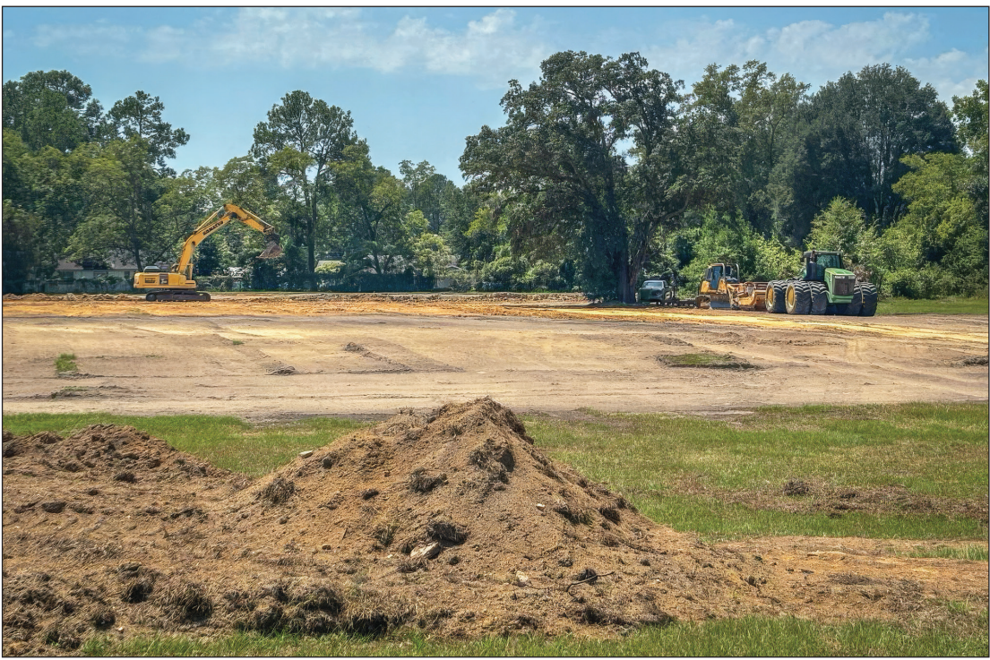
Staff Photo: Kathryn Crockett Construction continues on the South Madison Street-Alice Avenue drainage pond in Albany. City officials said Tuesday soil excavated from the site is being used at the nearby Henderson Gym project.
