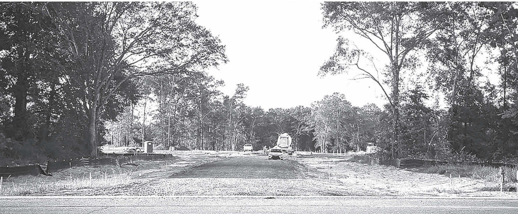
Site work is underway at 32 Crossing in Leesburg, where developers plan to begin construction with an initial 10 homes. The development could eventually include about 300 homes by the end of all development phases/KATHRYN CROCKETT
